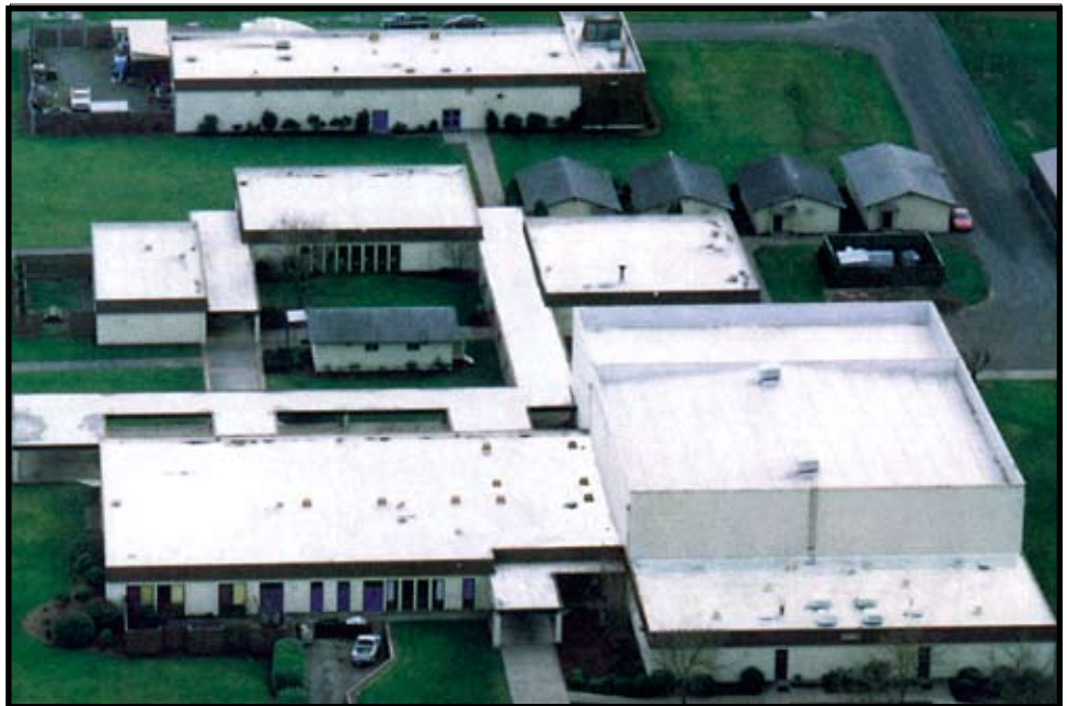
Harrisburg High School 550,000 sf 1st roof installed in 1979
